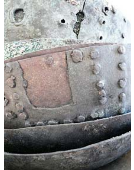
Riveted copper containers Photo : Jean-François REBEYROTTE
